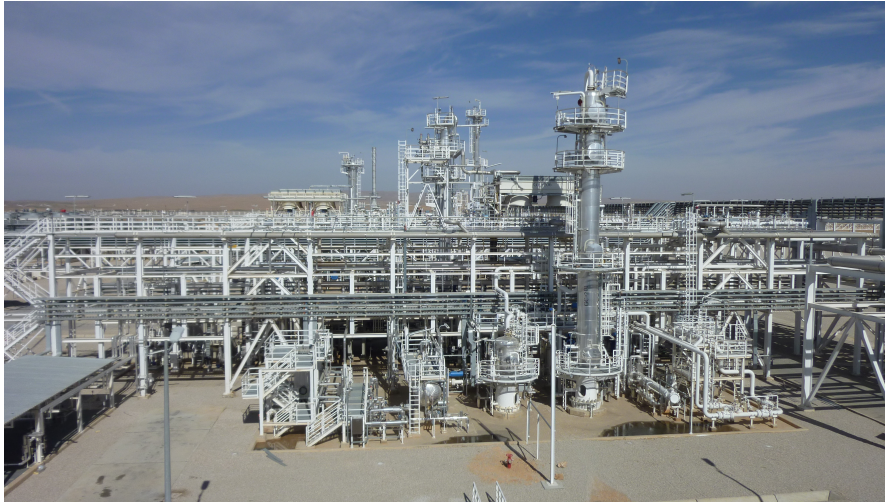
Figure 1: Natural gas processing plant (figure taken from [3] )
